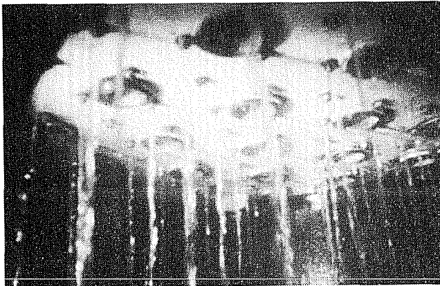
TUBED DRIP PAN IN SERVICE
